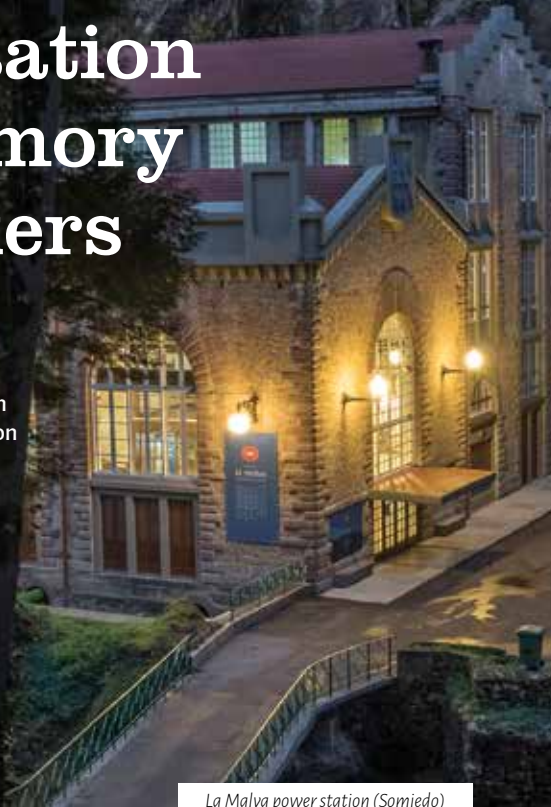
La Malva power station (Somiedo)
